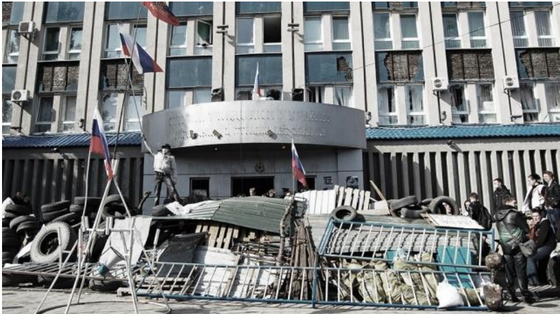
Building of the Security Service of Ukraine in Donetsk [98]
