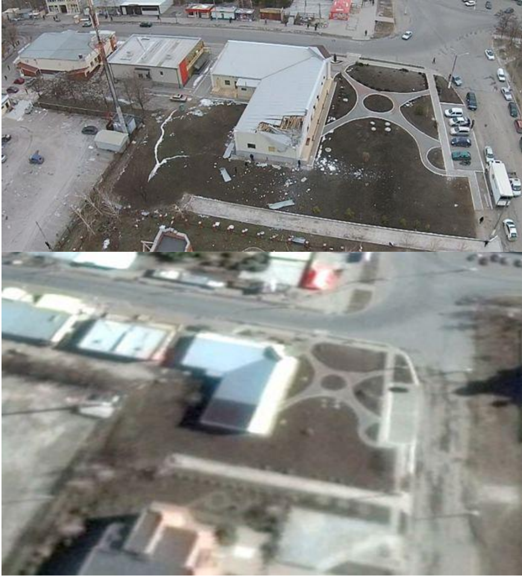
Top: a partly destroyed building from the drone footage, 24 January 2015; bottom: the same building restored, the darker area in the roof is the repaired part after the attack, 9 March 2015.
