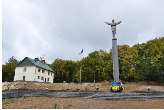
Figure 30. Column in Hurby with the Statue of Pokrova on the top and 33 crypts on the bottom of the column. The construction site for the monastery with one building already built to the left. Photo: Yuliya Yurchuk, October 2011.
